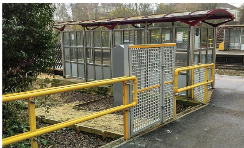
Gates Fences & Grilles
